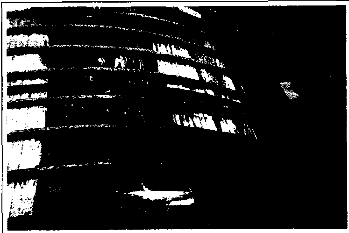
Deterioration of staves and bands
