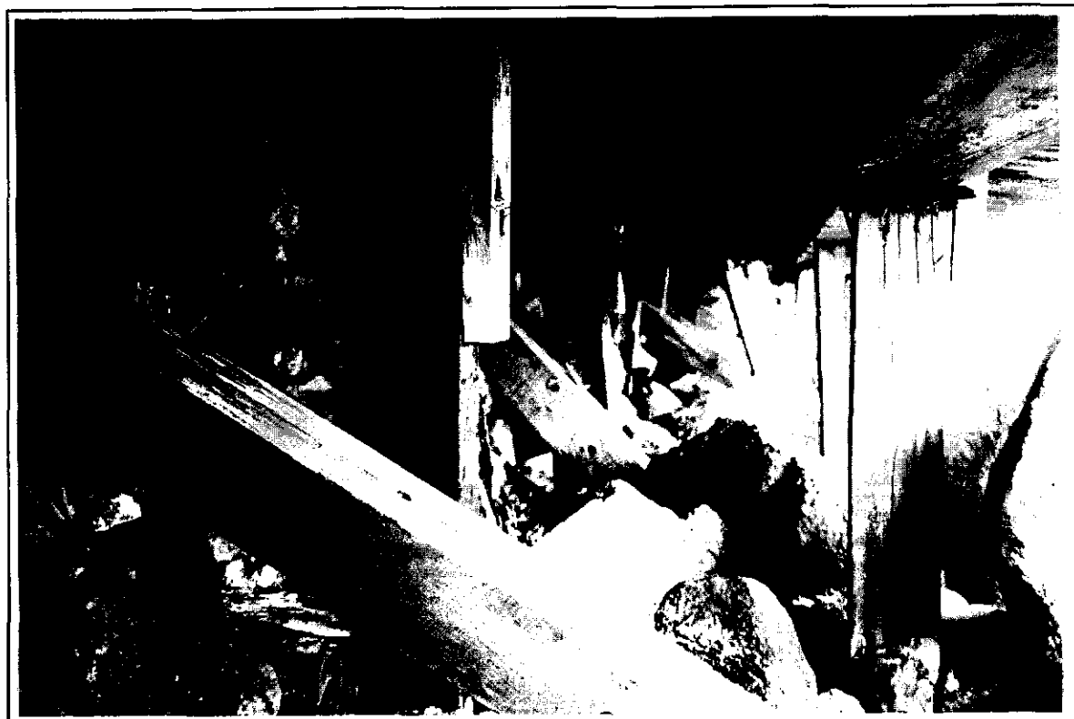
Rockfill and structural members below spillway apron
