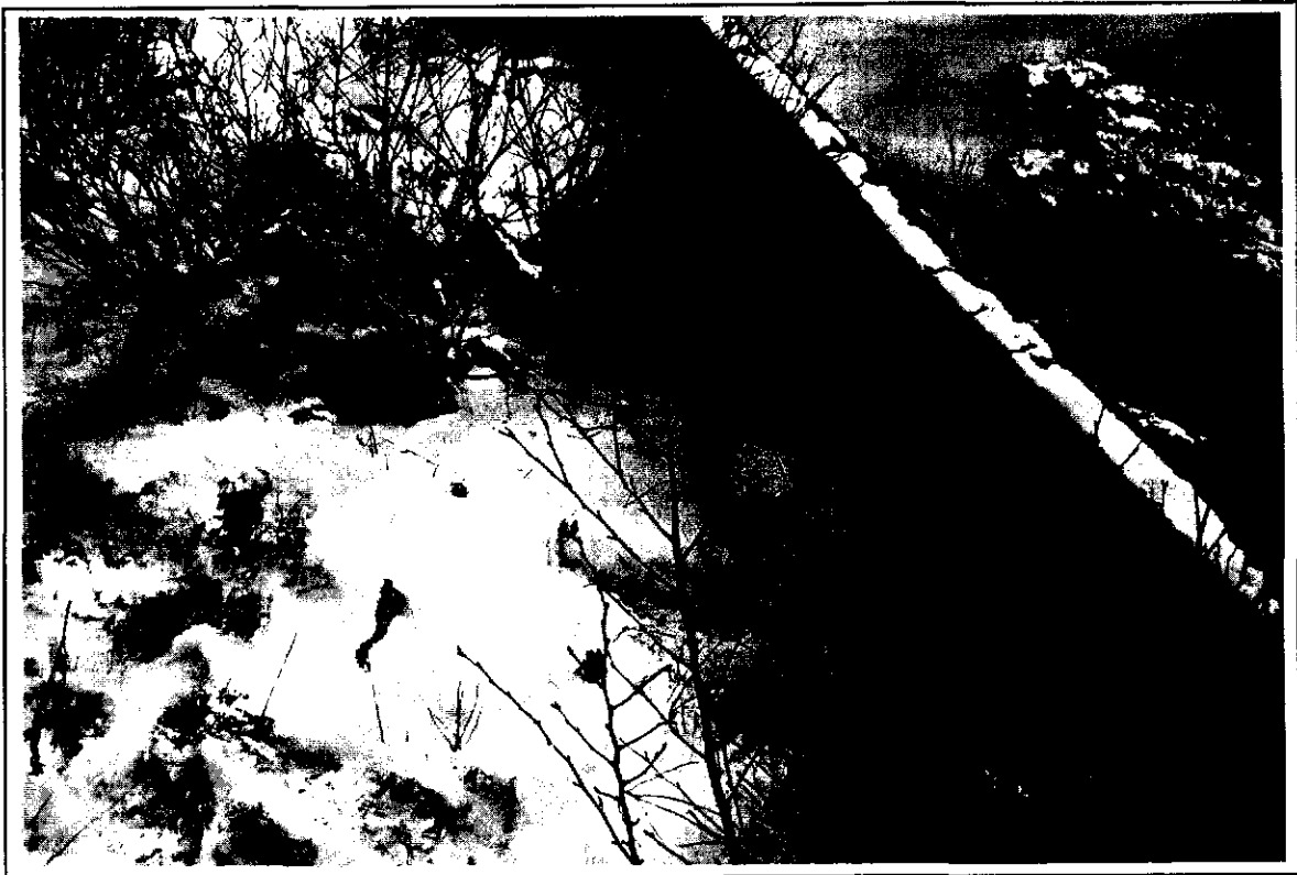
Settlement of crest beind cutoff wall
