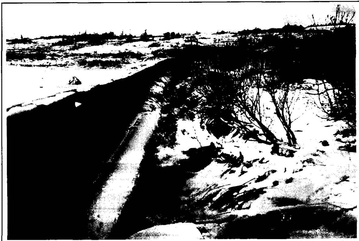
Settlement of crest beind cutoff wall
