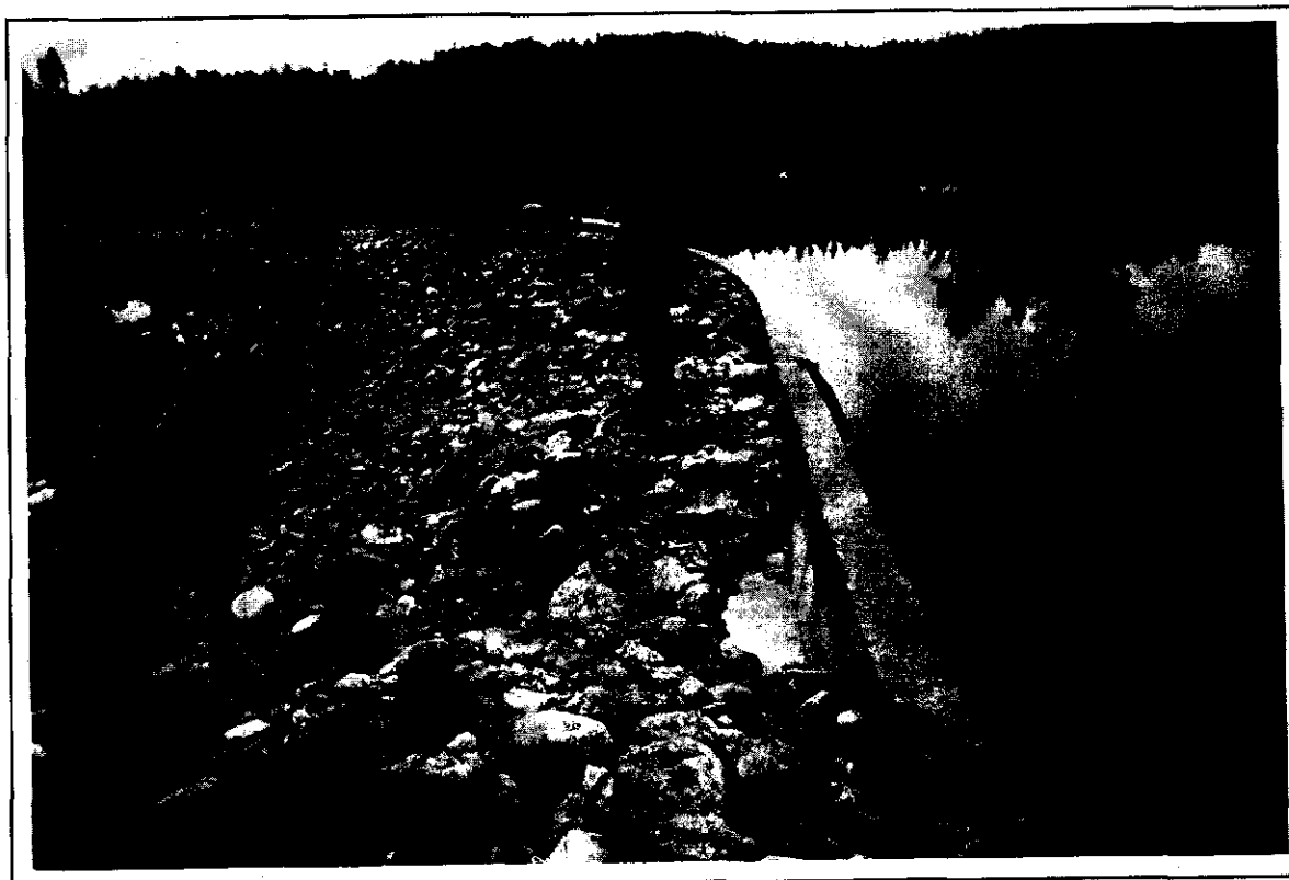
Erosion/settlement at crest
